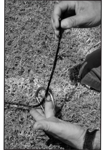
6. Feed tension line through ring in coil anchor
