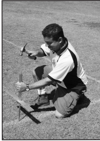
2. Hammer in ground stakes
