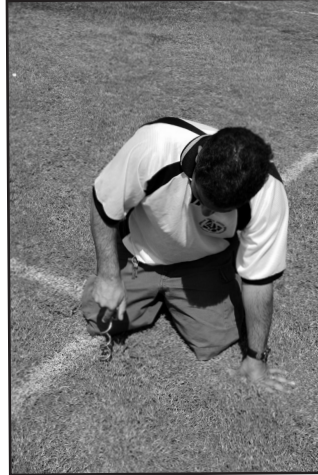
5. Screw in coil anchor approx. 3' from upright
